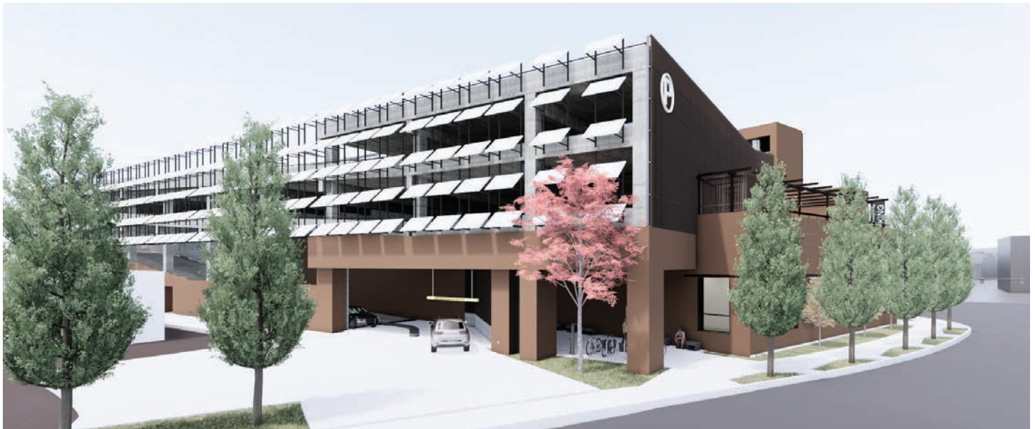
Rendering of the southeast corner of the building showing the solar photo-voltaic (PV) panels. The PV system will provide for approximately 18% of the building's power.
