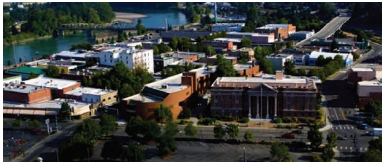
Aerial view of the project site from fundraising video
