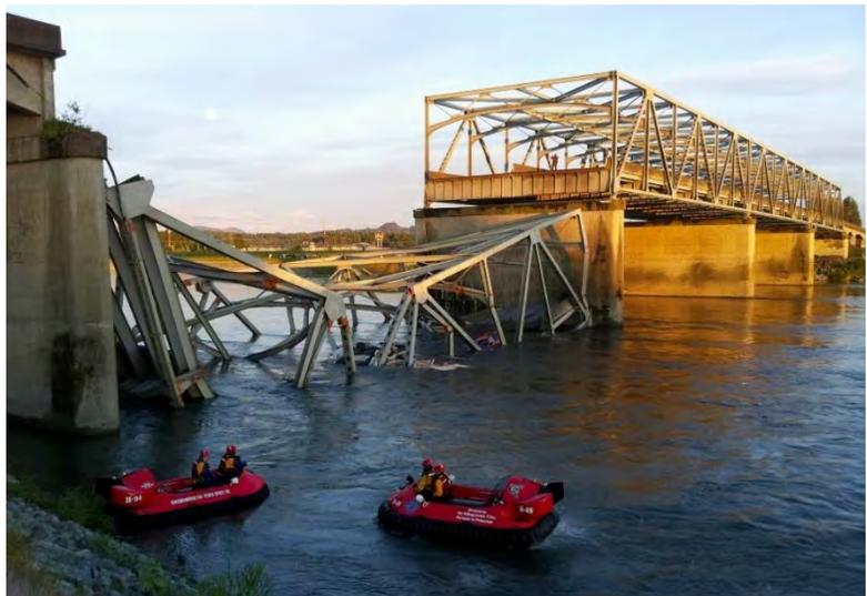
**Figure 3-8 Skagit County Bridge Collapse**
